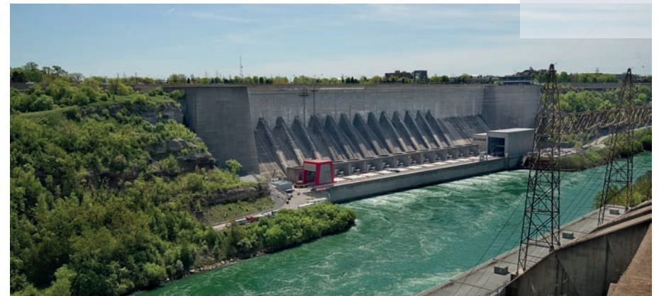
Adam Beck Generating Station © Robert Palmese
